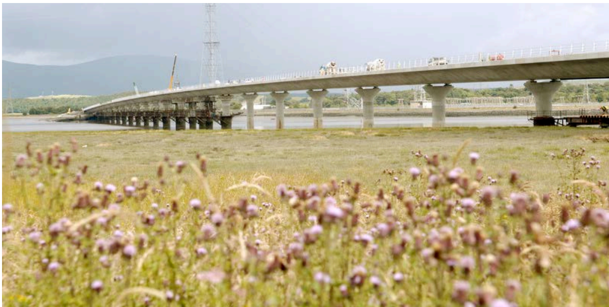
Bridge maintenance (courtesy of SEPA)
